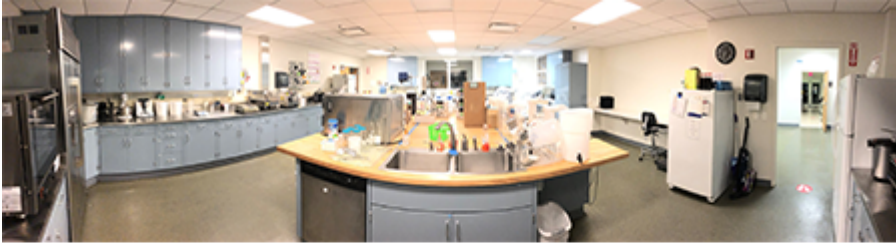
The food laboratory before the renovation
